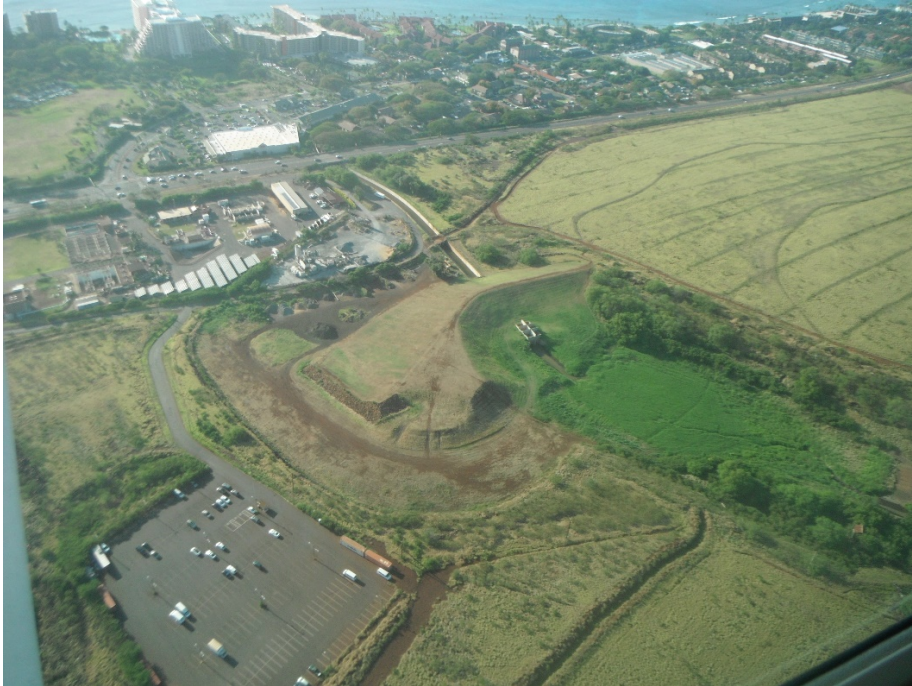
Photo 2-11: Aerial photograph of Honokowai Dam Structure #8
