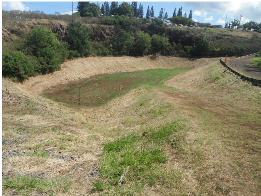
Photo 2-4: Looking upstream at Kaopala Basin
