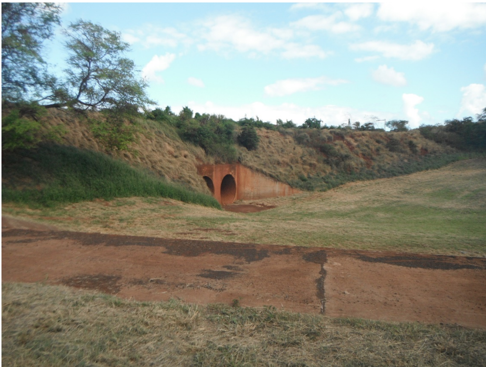
Photo 2-10: Mahinahina Basin, twin culverts under Honoapiilani Hwy
