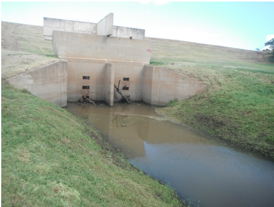
Photo 2-12: Honokowai Intake Structure
