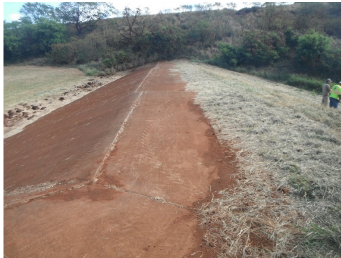
Photo 2-8: Mahinahina Basin, Looking northeast from the top of the embankment
