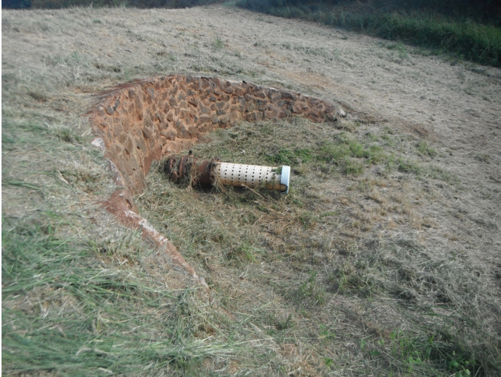
Photo 2-9: Mahinahina Basin, inlet pipe
